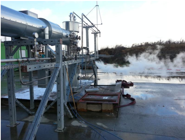
Impressions from the pumping test
